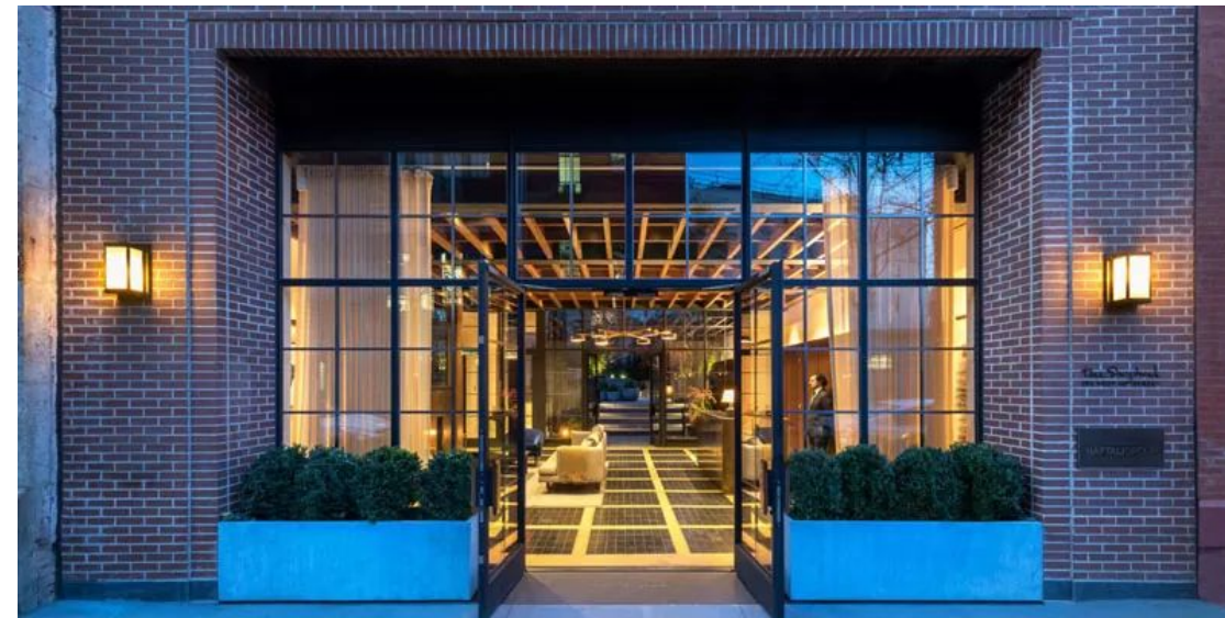
Example of brick return conditions
