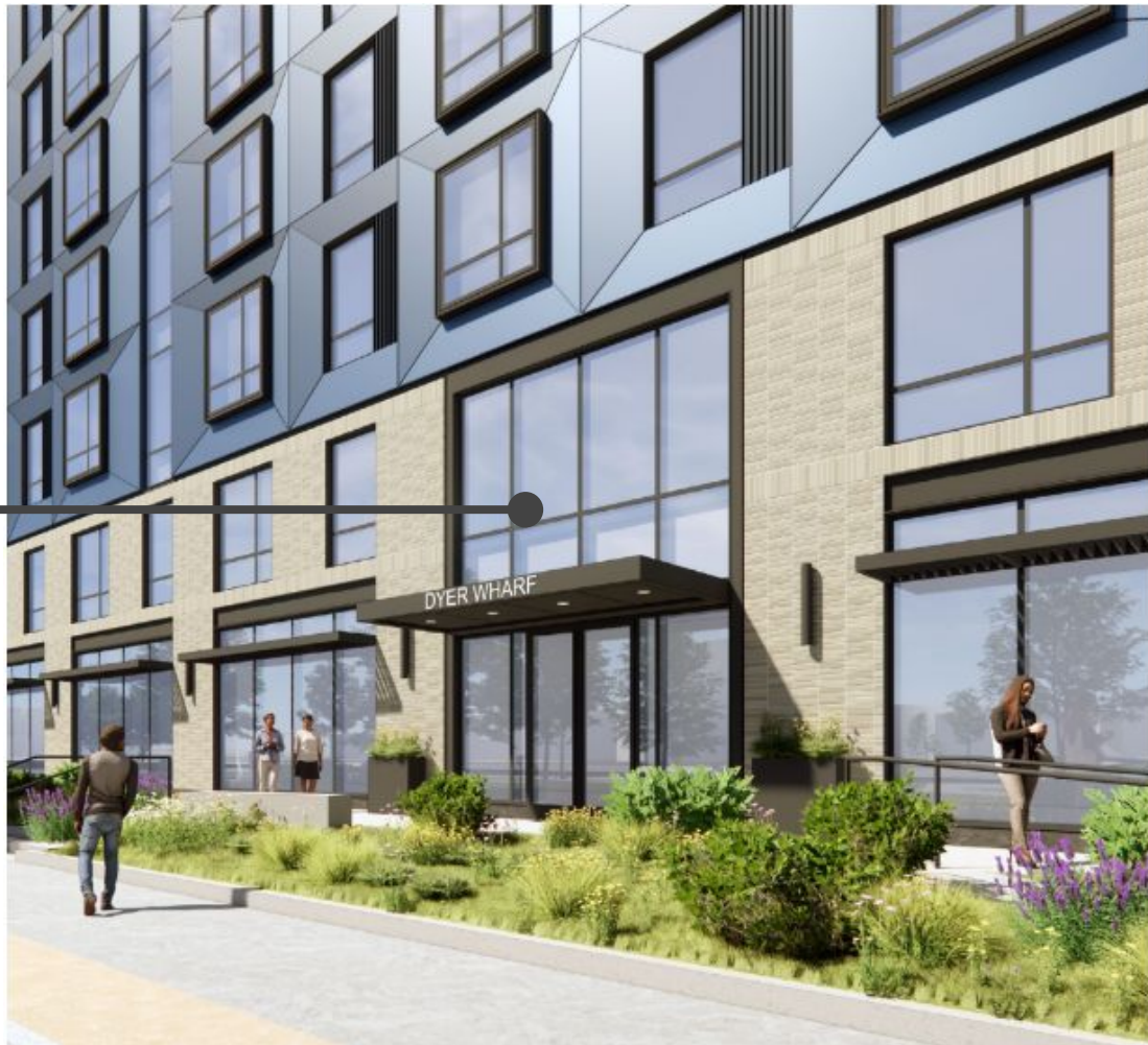
VIEW OF MAIN ENTRY FROM PECK STREET
